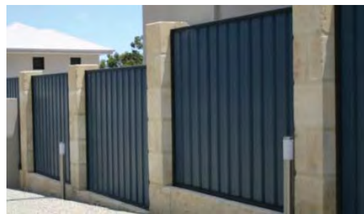
Fence Type 1 Sandstone Post with Colourbond panels
