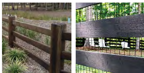
Fence Type 3a 1.2 Estate fence-Post & rail (three) fence (colour dark grey/black) with wire mesh fixed to rear face (removing scalability)
